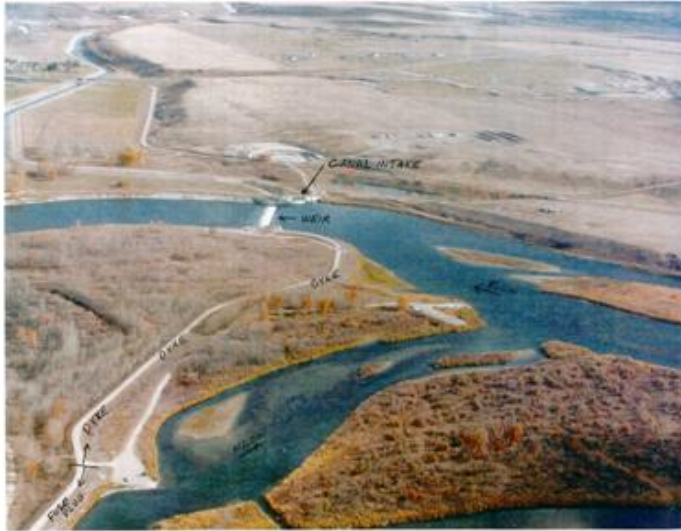
Figure 15: Aerial photograph of Carseland diversion showing dike across Johnson's Island
