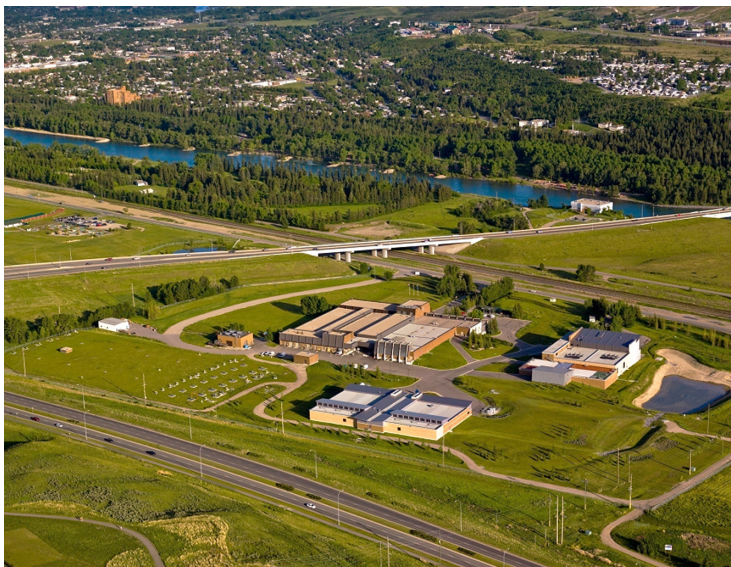
Bears paw Water Treatment Plant, Calgary
